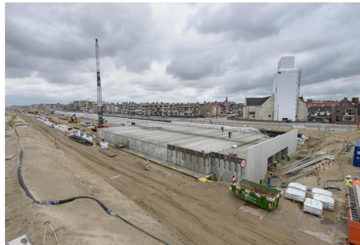
Multifunctional dykes: innovative space-saving solutions: construction of an underground car park within the dyke at Katwijk.
